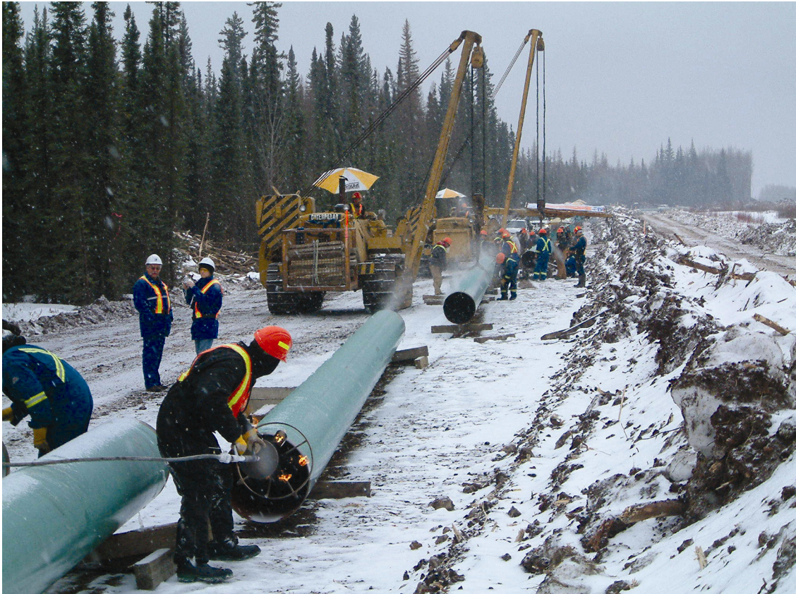
Pipeline being constructed near Wabasca, Alberta
