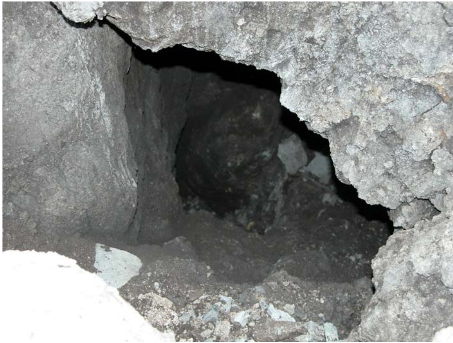
Photo 3: Close-up of the small opening or tunnel shown in Photo 2. The tunnel extended downward for at least another 2 metres by estimation.
