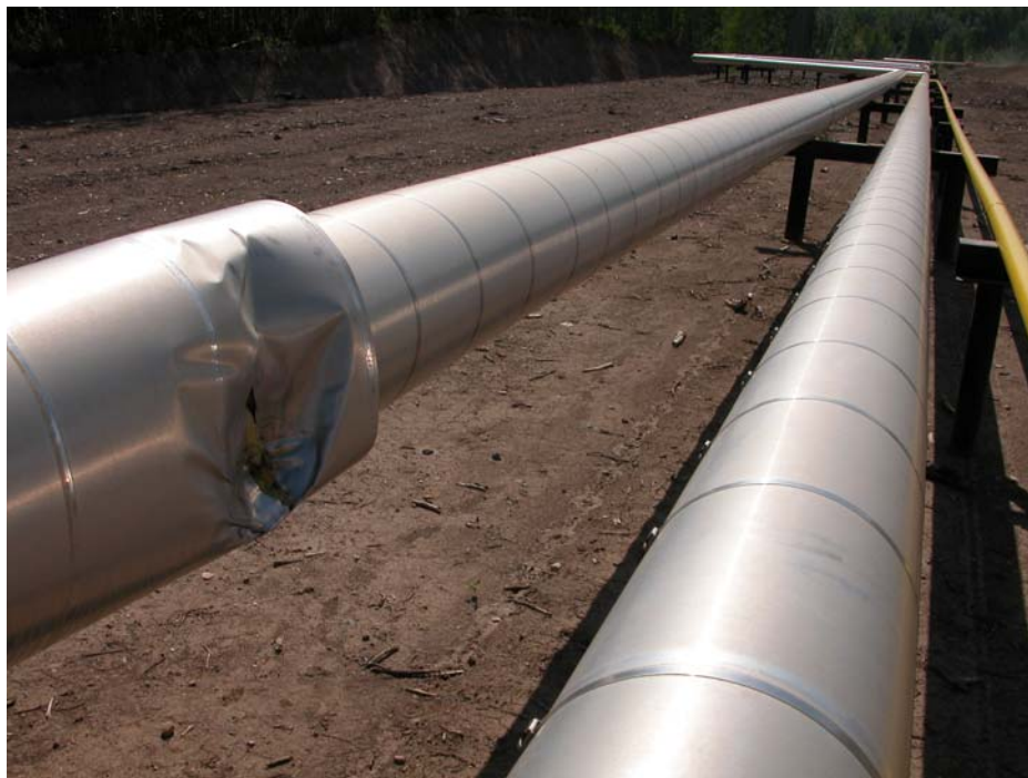
Photo 40: Pipeline impact looking south toward the plant.
