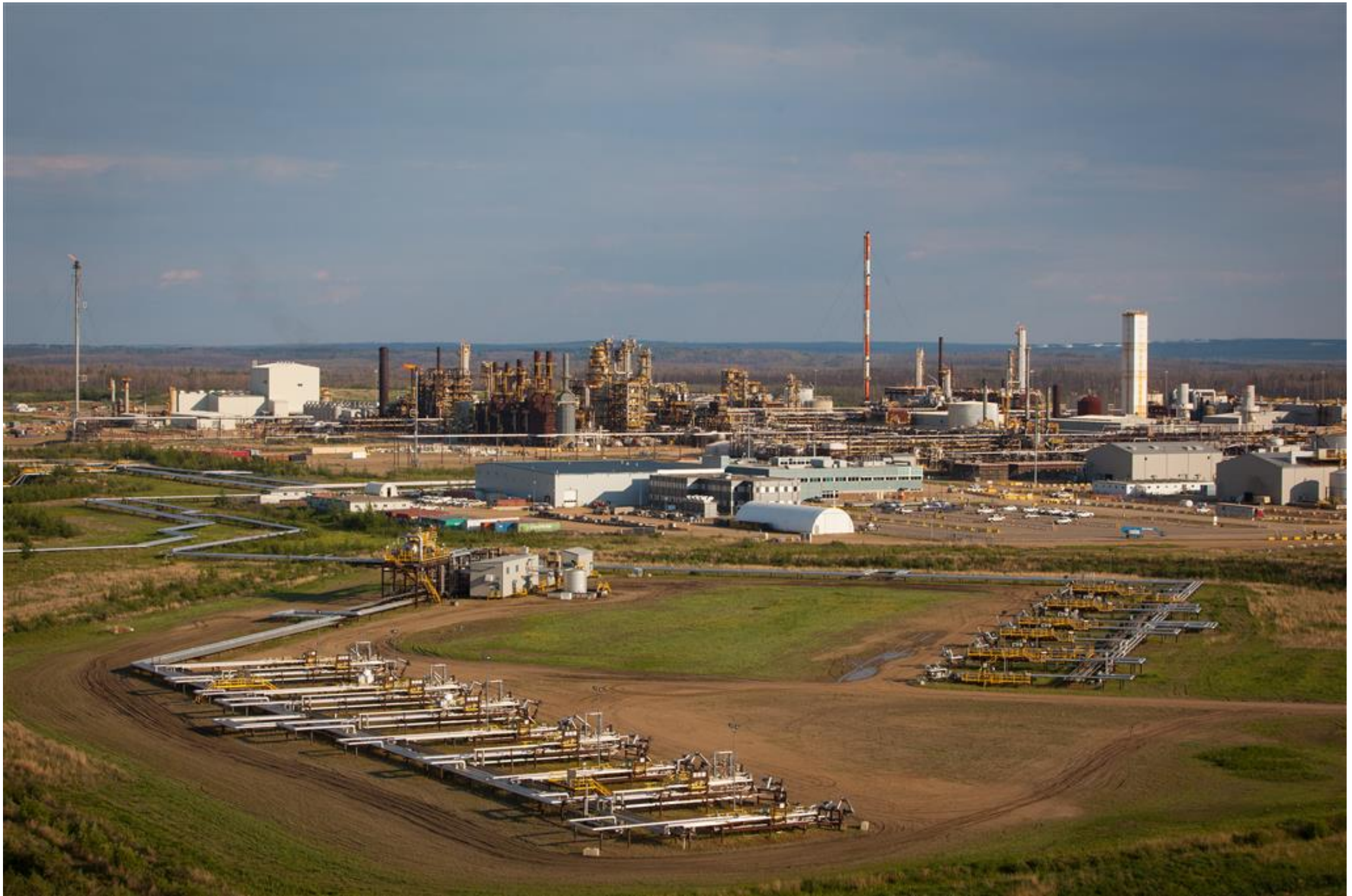
Long Lake facility overview with Pad 9 in the foreground - June 19, 2018
