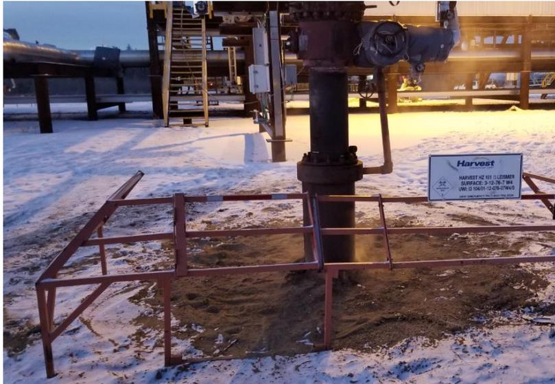
**101 Pair 3 injector - bare dual string completion**
