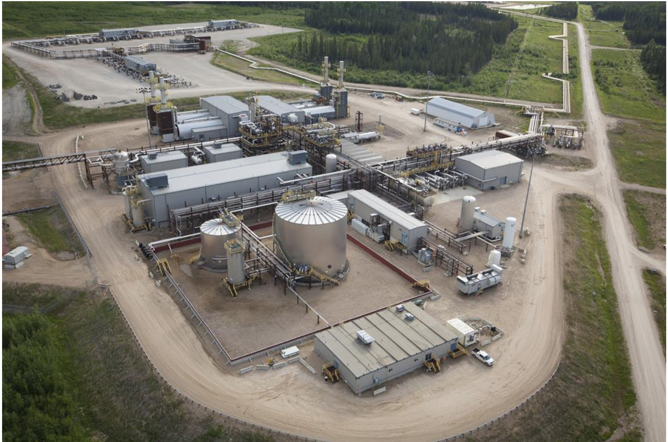
Aerial of K1A Steam Generation Facility with Well Pad 2 in the background – June 19, 2018
