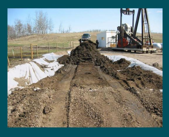
Properly constructed Biopile- bermed with a liner for run-on and run-off control
