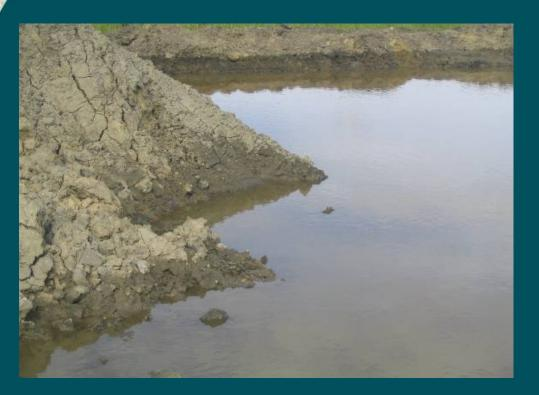
Underground tank failed the integrity test. Licensee excavated tank and removed contaminated soil. The contamination had migrated and impacted a large area, approximately 1000 m³ of contaminated soil removed and there is evidence that the groundwater was adversely impacted. This is a reportable spill.
