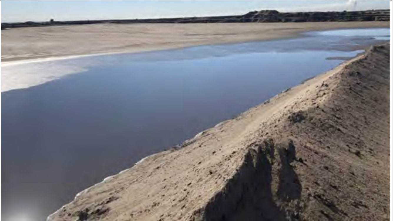
Photo 07 – South view of partially drained deposited AFD on ETF.
