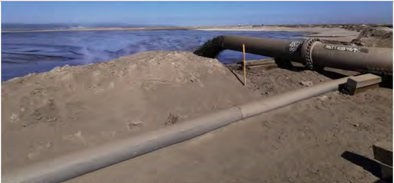
Photo 03 –View of active discharge line NST 1, beach development.
