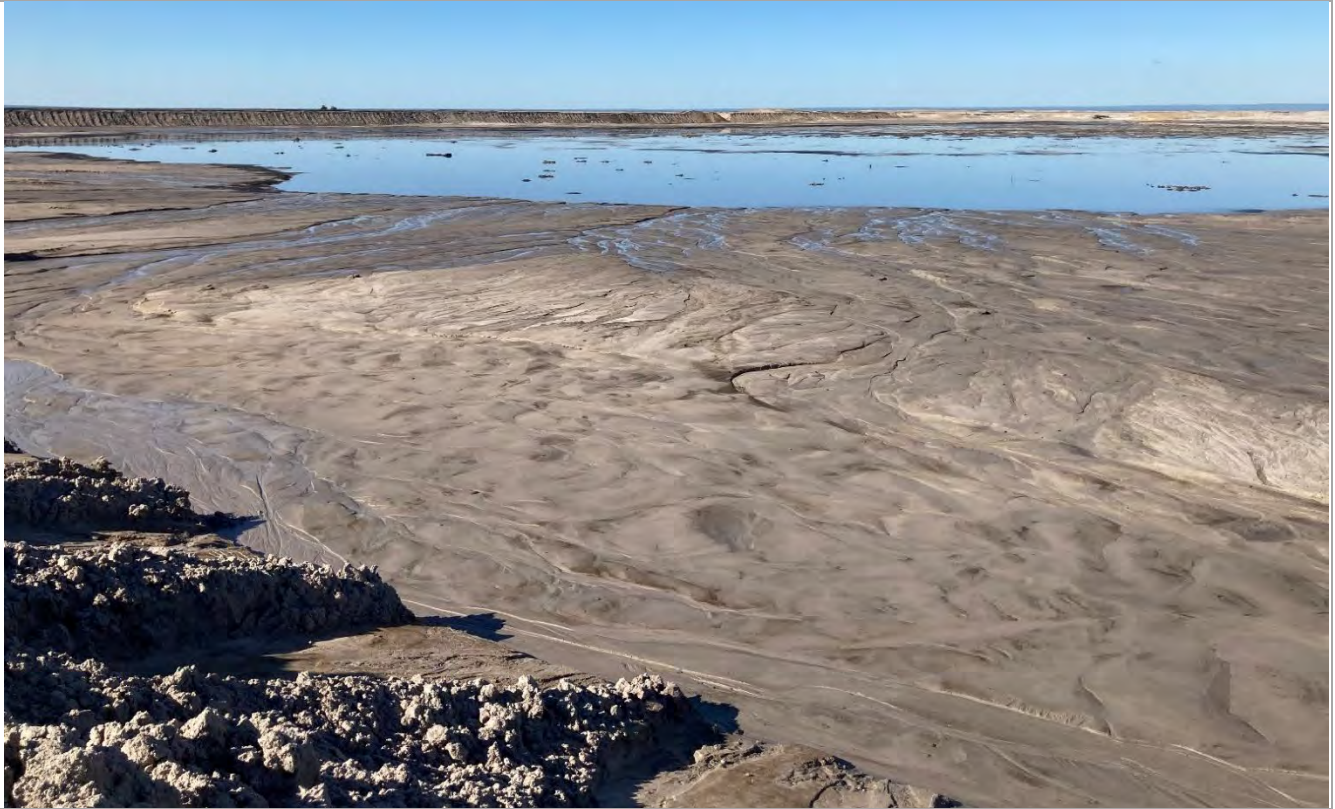
Photo 03 – South view of ETF treated tailings deposit BAW beach development due to infilling.
