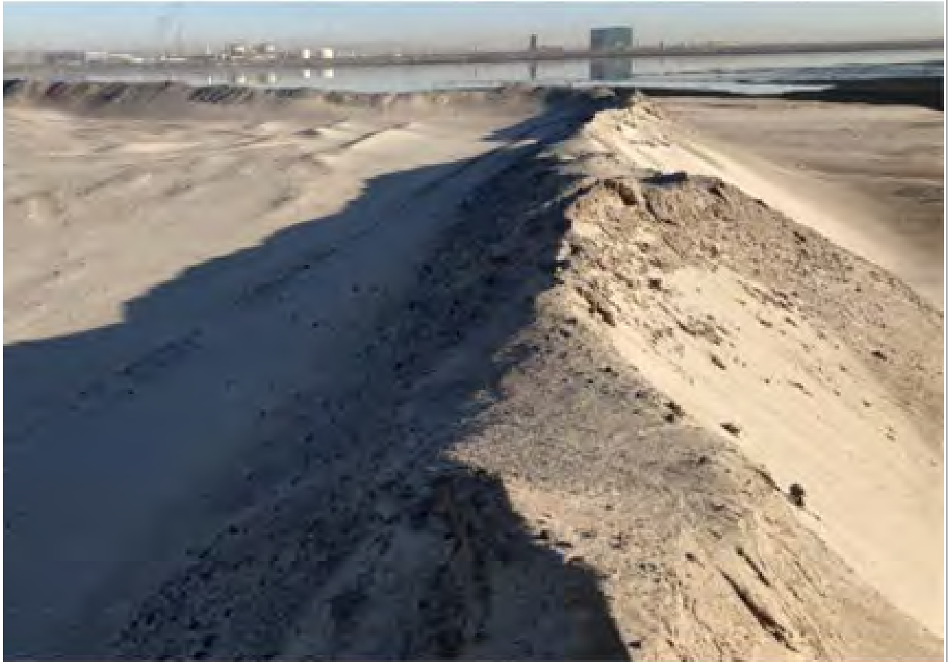
Photo 13. North view from IPC 3 peninsula showing 5 m elevation of Blanket Cap layer.
