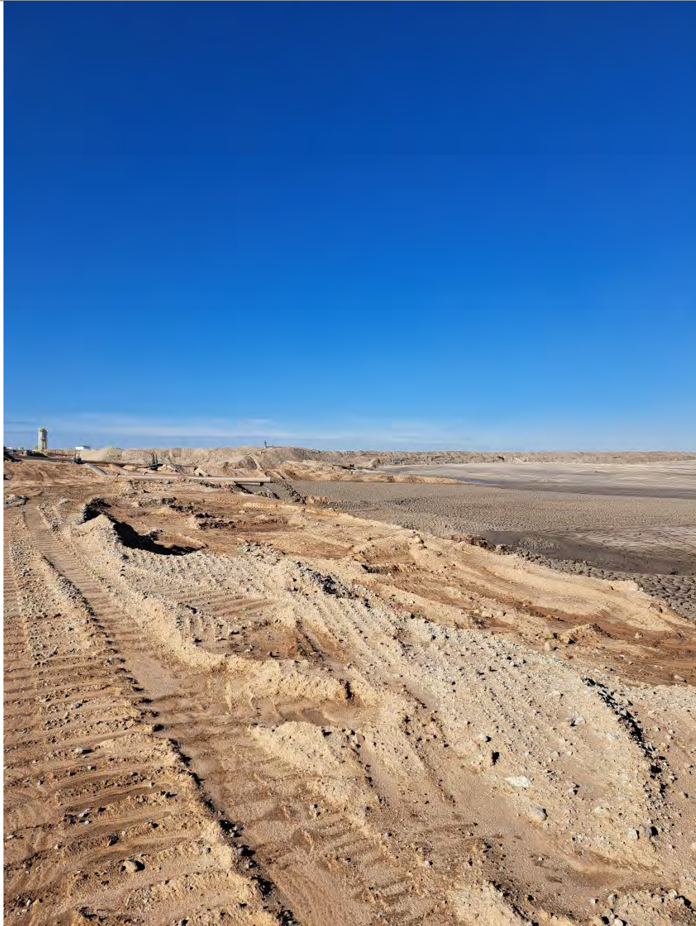
Photo 02 – CST beach on TT deposit in background, desiccated TT deposit in foreground
