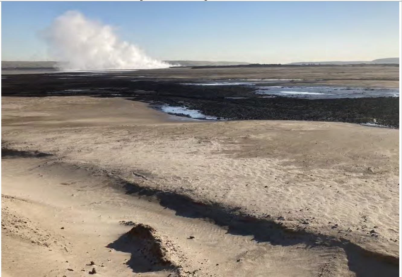
Photo 12 – Northeast view from CST peninsula in IPC 3 showing active deposition and bitumen collection along mixed deposit beach.
