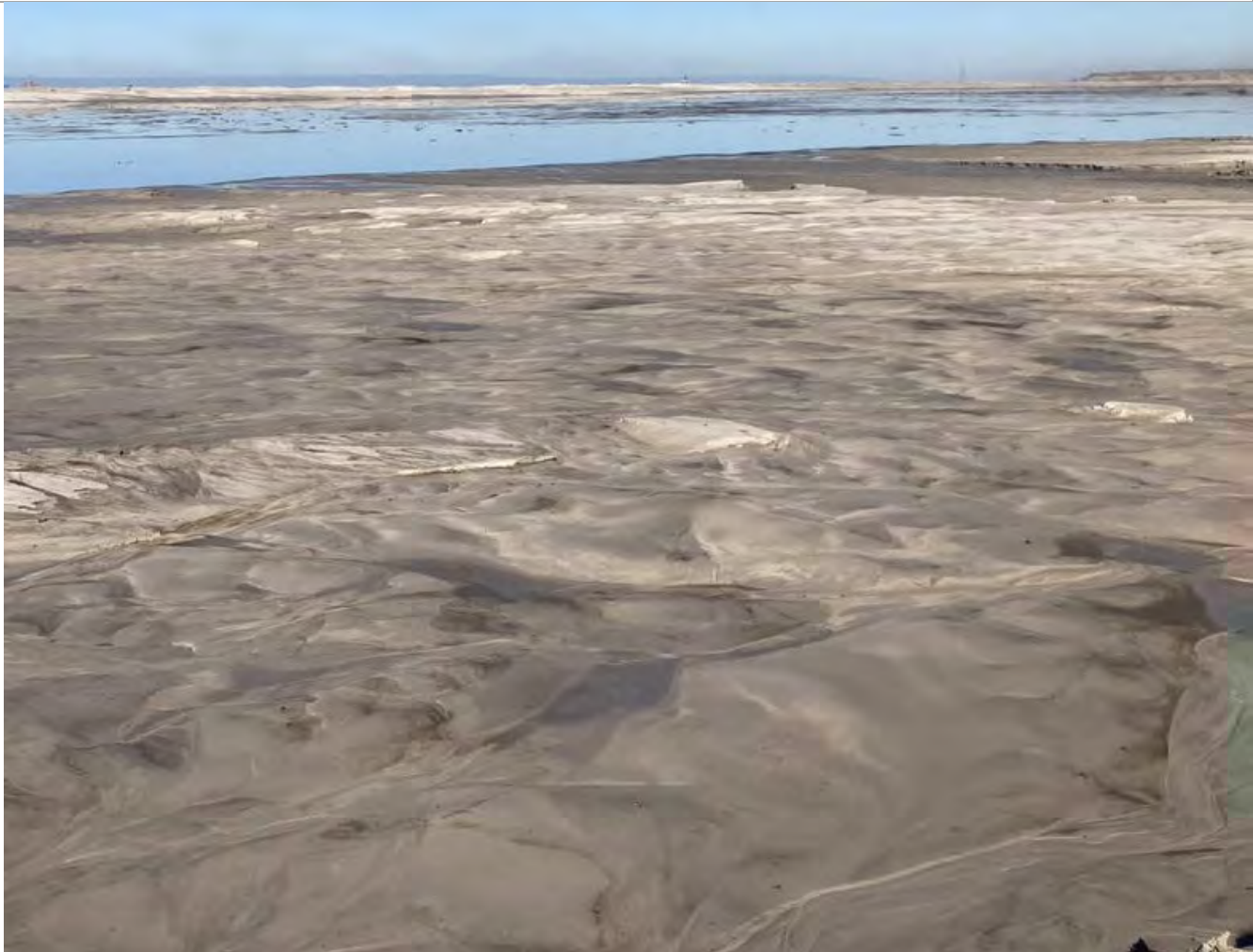
Photo 02 – North view from the south end of ETF treated tailings deposit BBW pushed to surface due to infilling.
