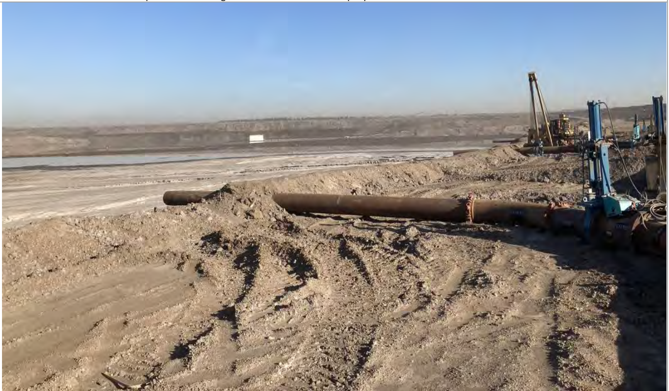
Photo 14. Northeast view from East side of IPC 4 showing establishment of deposition lines.
