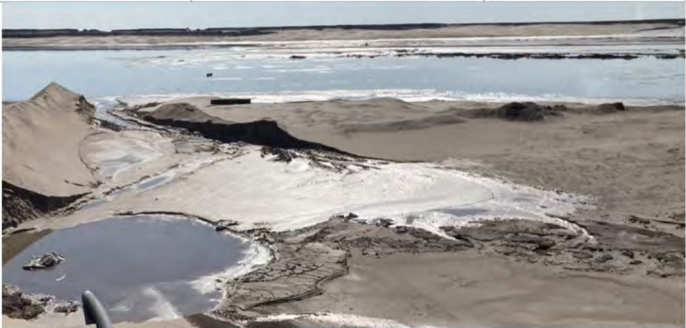
Photo 01 – South view of over-topped splitter dike between ETF / DDA1 and SC 1.
