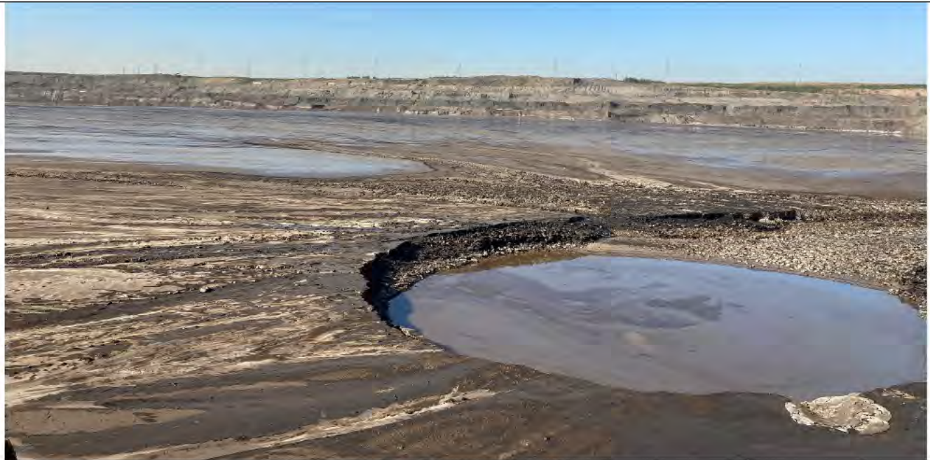
Photo 05 –View of active discharge line NST 3, beach development, presence of bitumen and gravel.
