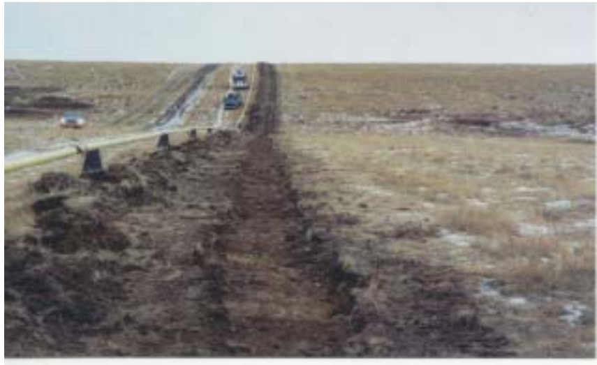
Photo 32 Partial sod salvage in shallow topsoils
