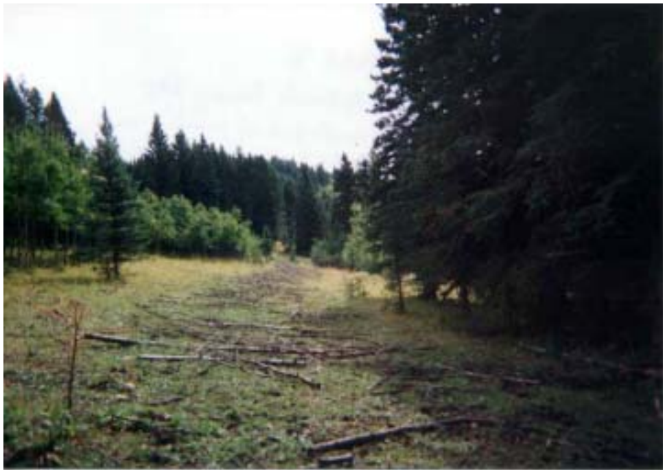
Photo 42 Aspen, salvaged from clearing operations, was used to control erosion on this natural recovery site.
