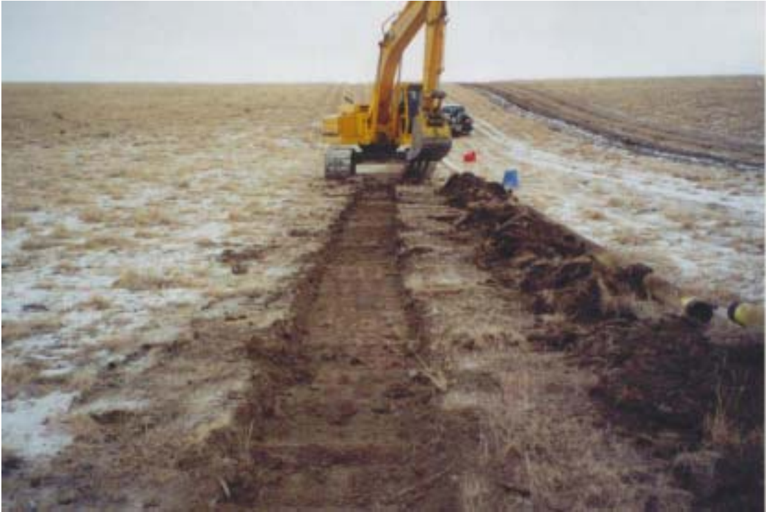
Photo 29 Trench line stripping in frozen ground conditions
