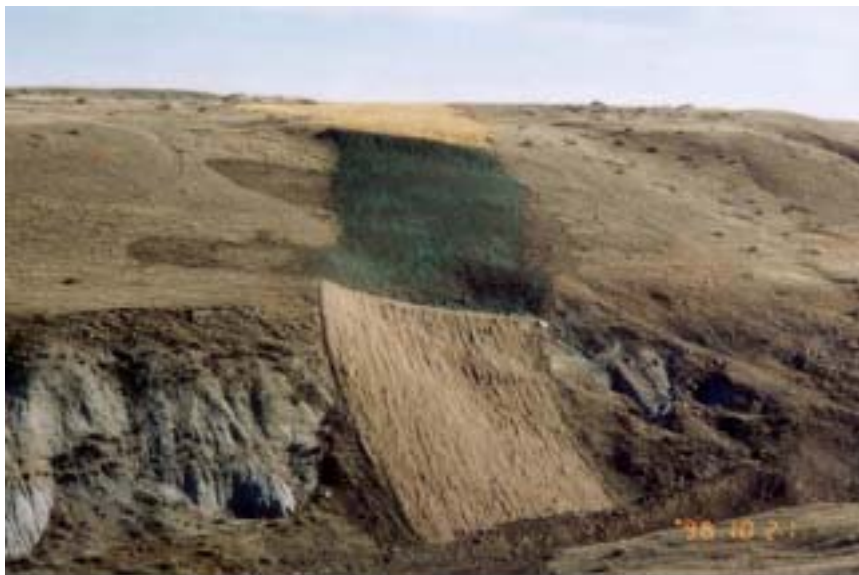
Photo 41 Erosion control options: erosion control fabric, hydromulch and straw crimping
