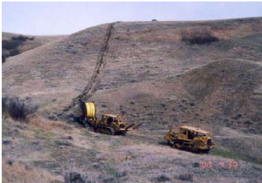
Photo 18 Minimizing disturbance with small diameter pipe
