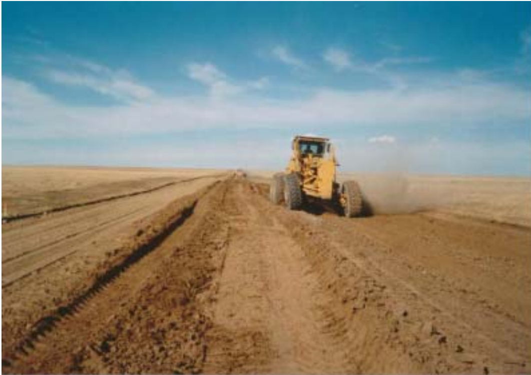
Photo 28 Double blade width stripping
