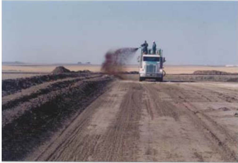
Photo 26 Applying soil tackifier to prevent wind erosion
