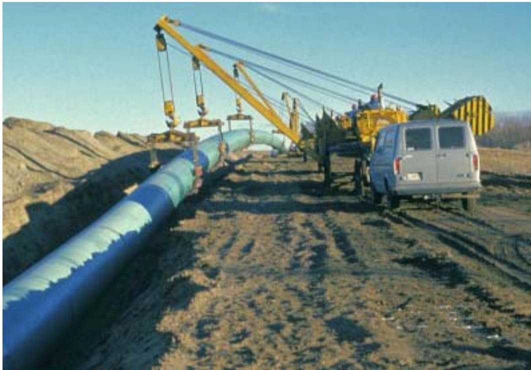
Photo 16 Lowering in large diameter pipe.
