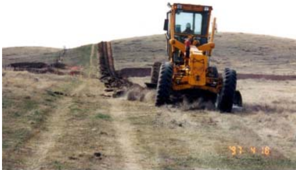
Photo 27 Blade width stripping
