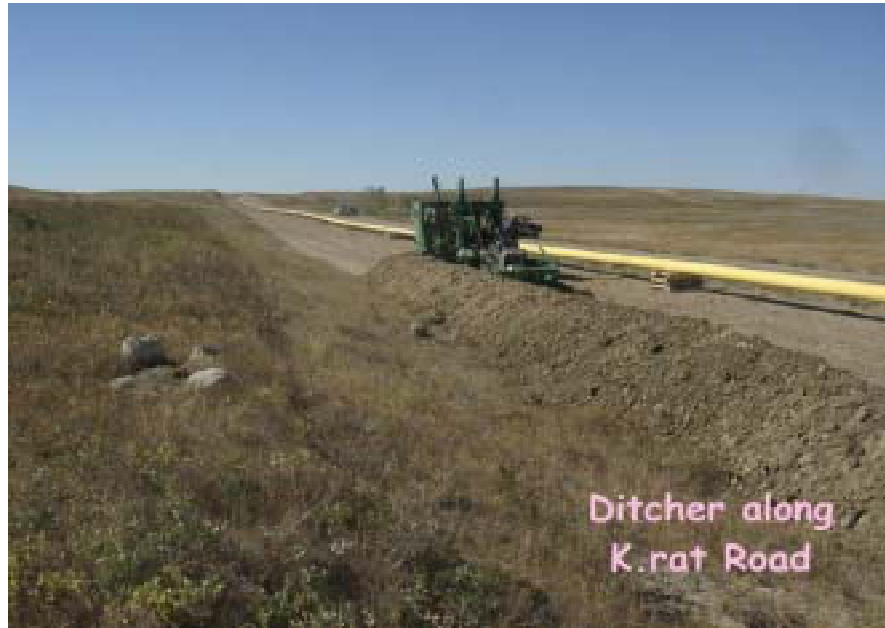
Photo 17 Minimizing disturbance with mid-sized pipe (16 inch pipe)
