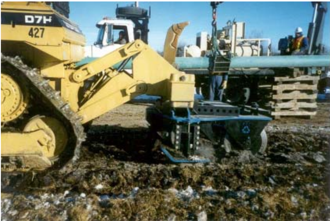
Photo 49 Frozen topsoil cutter mounted on a dozer.
